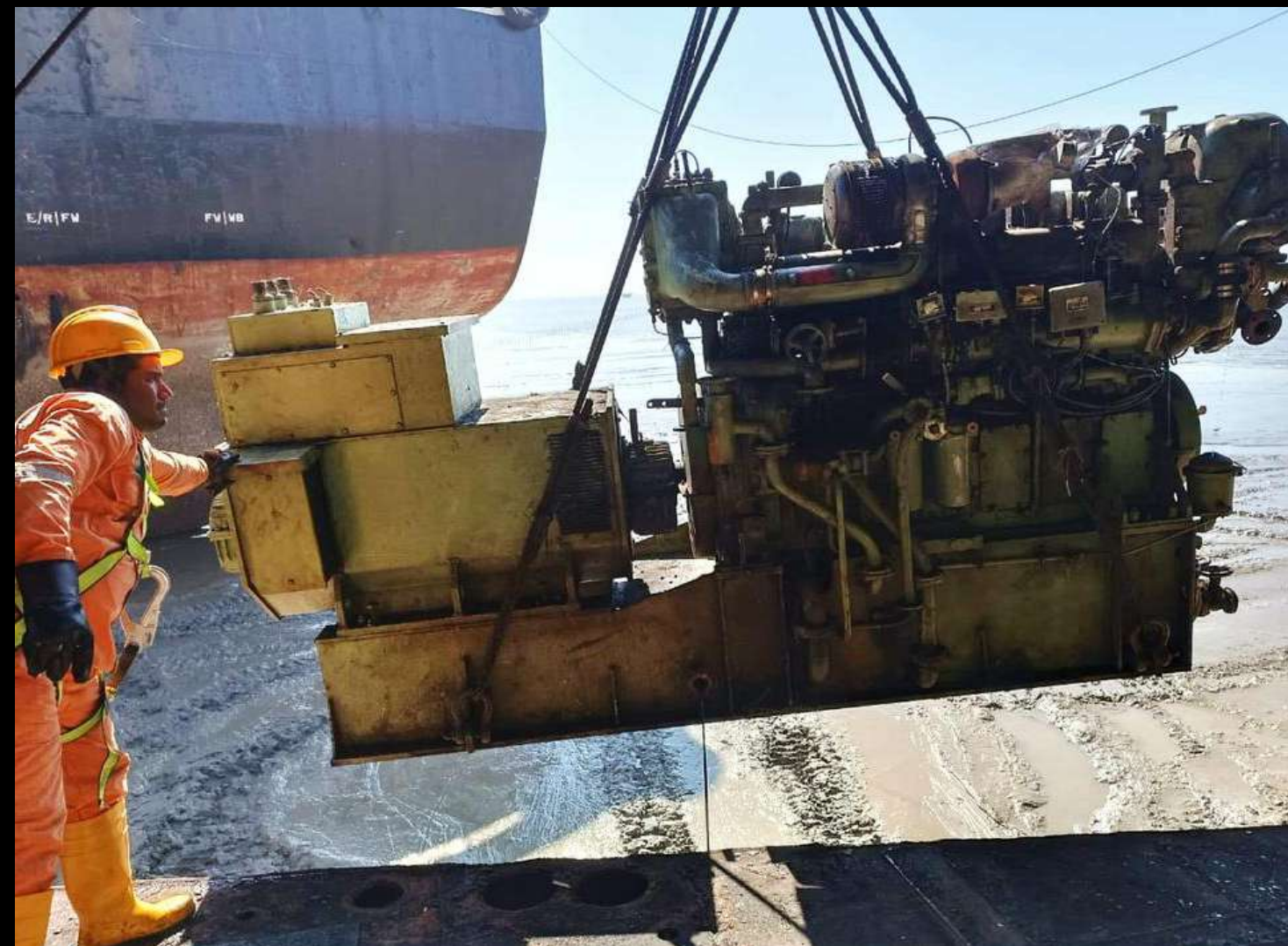
OUTFITTING REMOVAL PROCESS FROM SHIP
